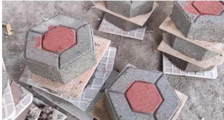
Gambar 6. Proses Pencetakan Paving Block
