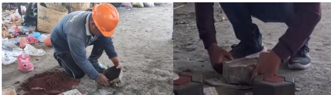
Gambar 5. Proses Pencetakan Paving Block
